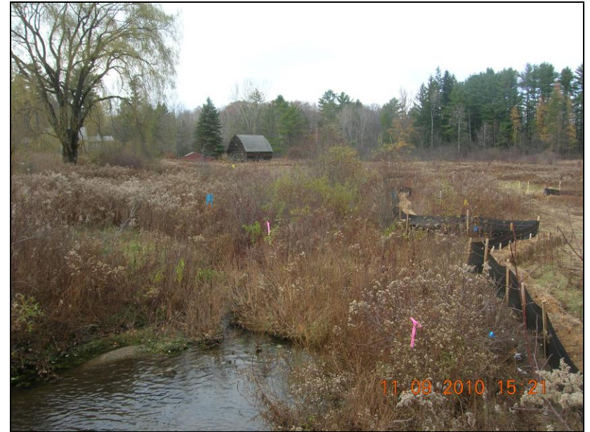
Wetland Restoration: Site Preparation November 2010
