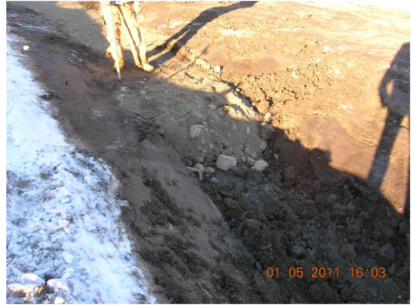
Wetland Restoration: Gravel Substrate Installation January 2011
