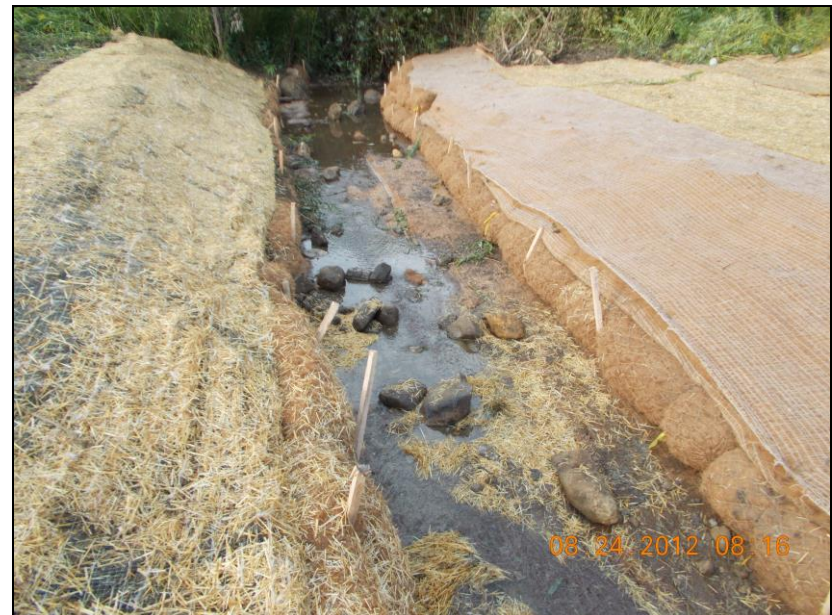
Wetland Restoration: Channel Connection and Water Release August 2012
