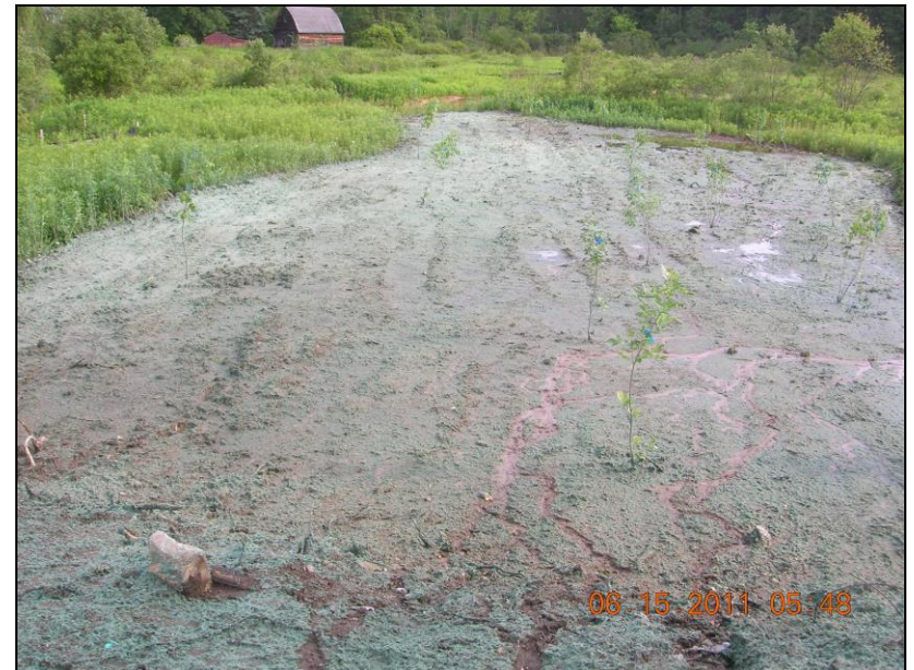
Wetland Restoration: Final Hydro-Seeding June 2011
