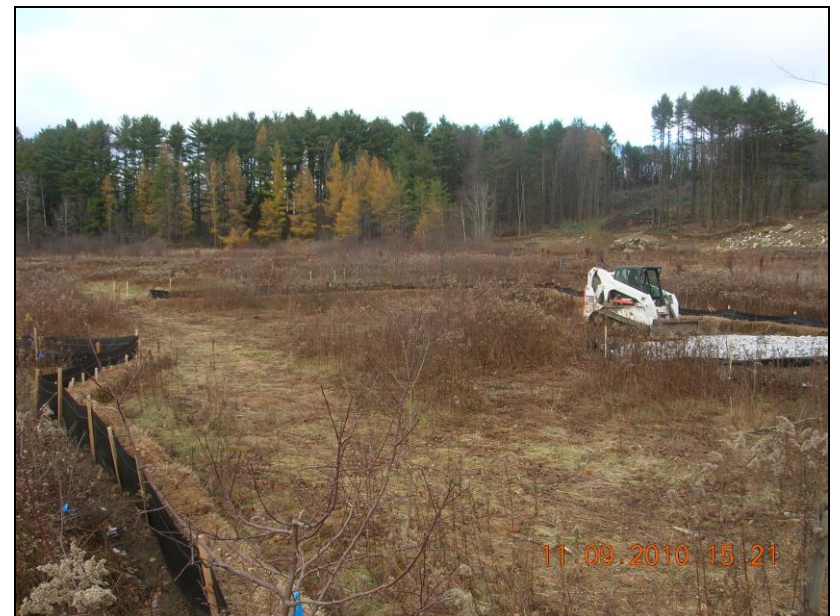
Wetland Restoration: Site Preparation November 2010
