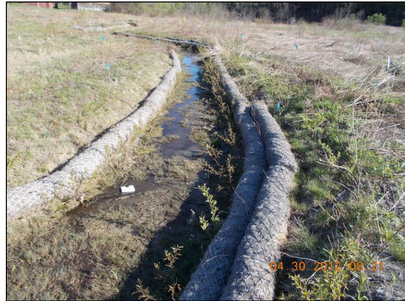
Wetland Restoration: April 2012
