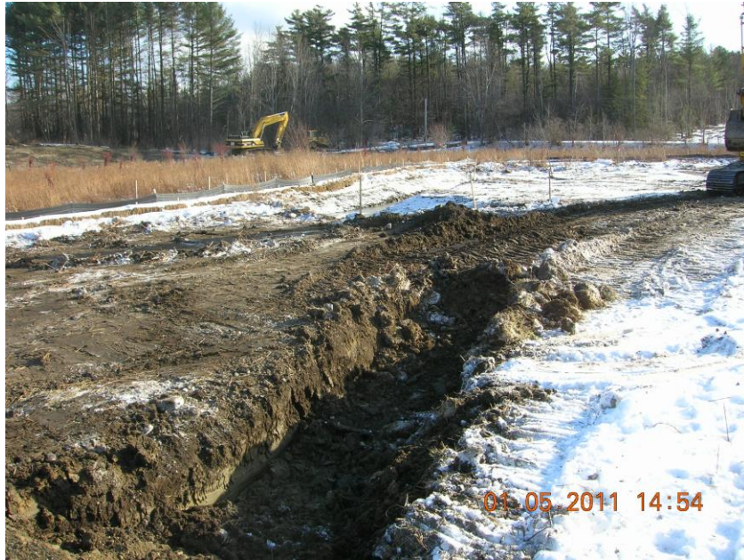
Wetland Restoration: New Channel Excavation January 2011
