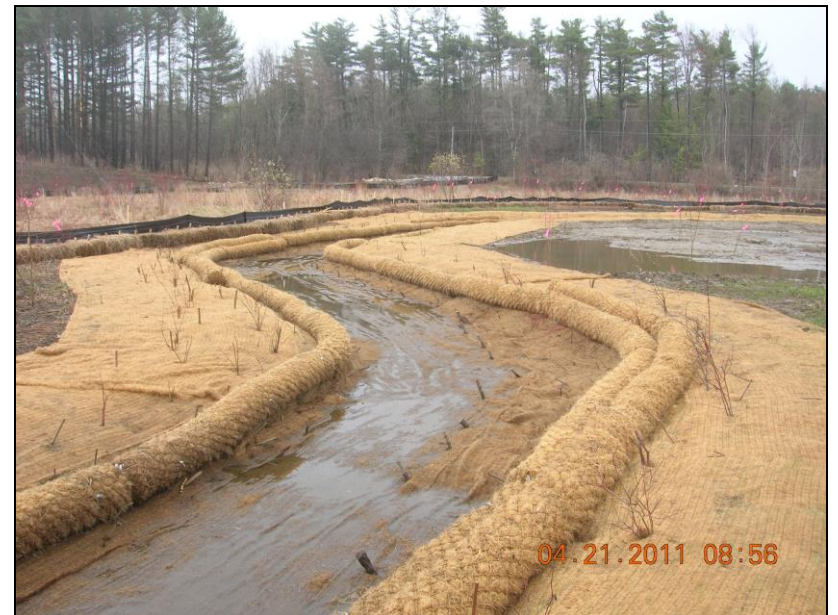
Wetland Restoration: Channel Construction/Stabilization April 2011
