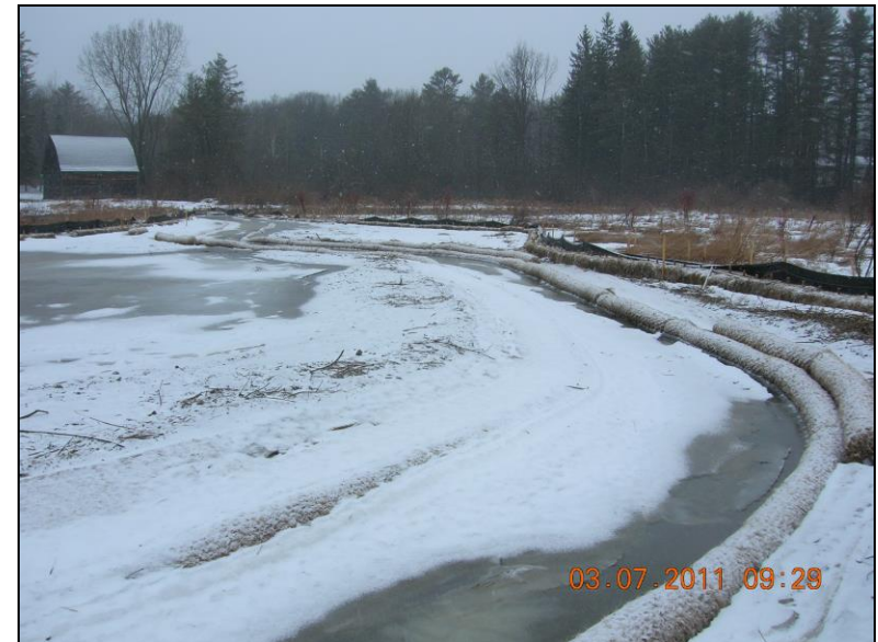
Wetland Restoration: Channel Construction March 2011
