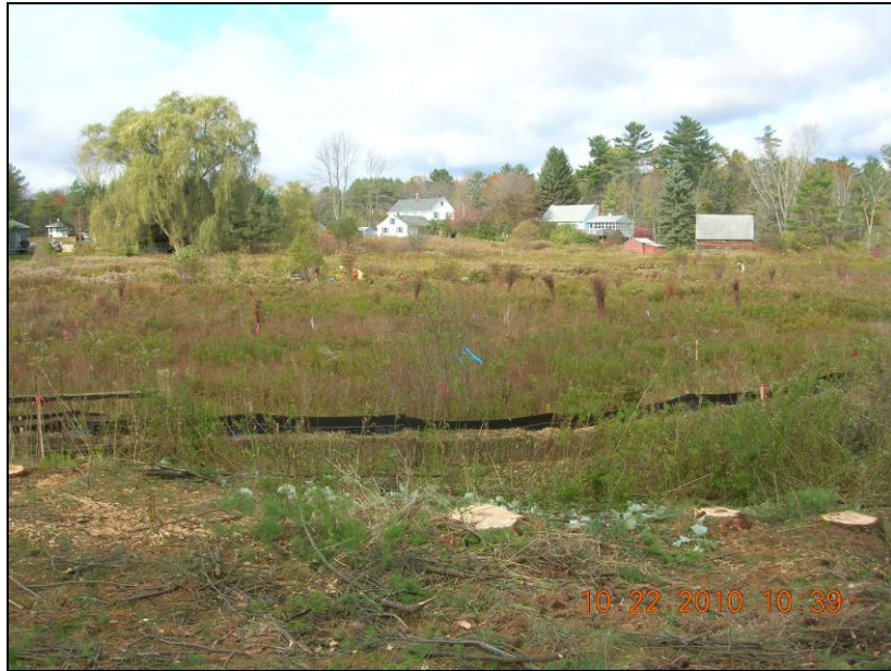
Wetland Replication: Site Preparation October 2010
