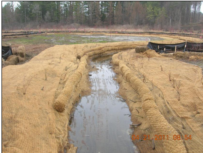
Wetland Restoration: Channel Construction/Stabilization April 2011
