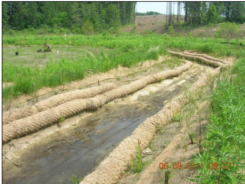
Wetland Restoration: Planting (willow stakes along channel) June 2011
