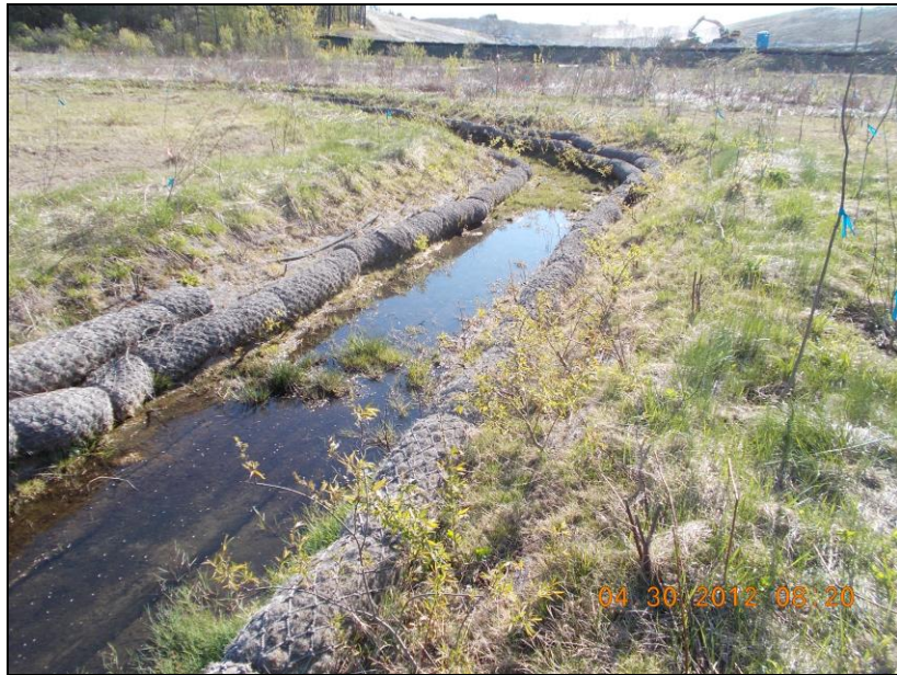
Wetland Restoration: April 2012
