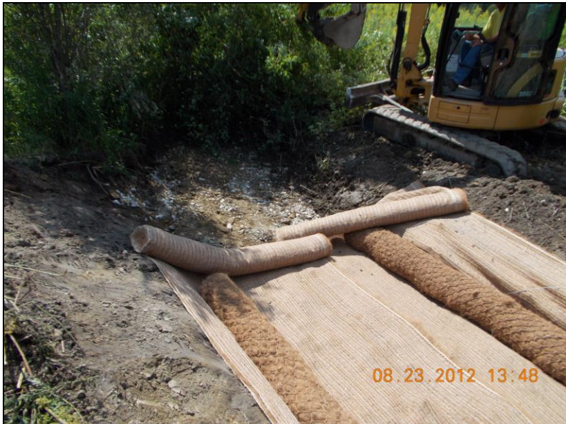
Wetland Restoration: Channel Stabilization August 2012
