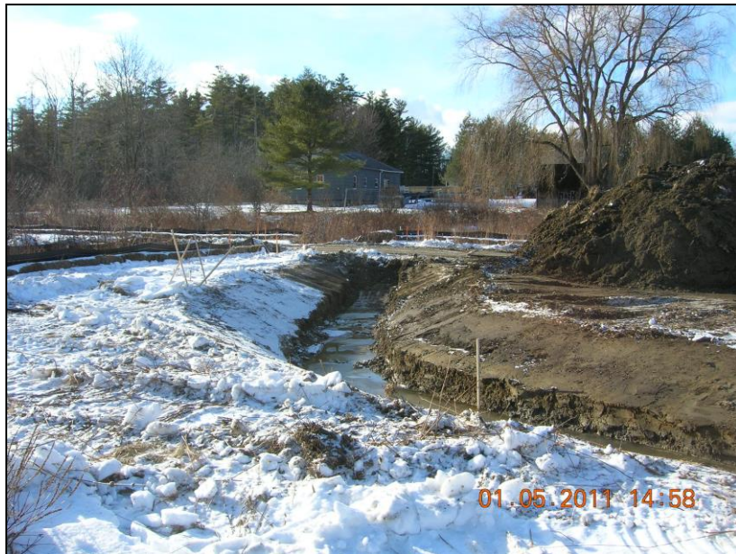
Wetland Restoration: Channel Construction January 2011
