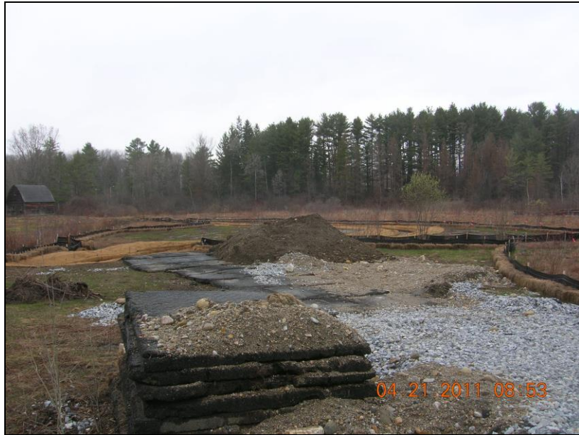
Wetland Restoration: Channel Construction April 2011
