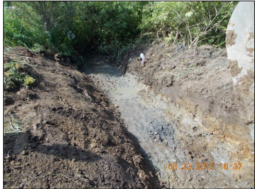
Wetland Restoration: Creating Channel Connection August 2012
