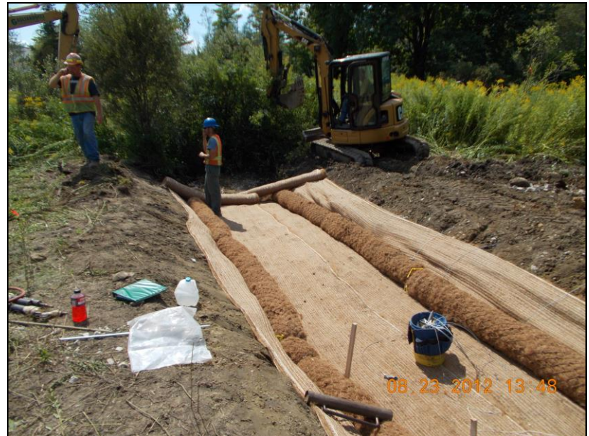
Wetland Restoration: Channel Stabilization August 2012
