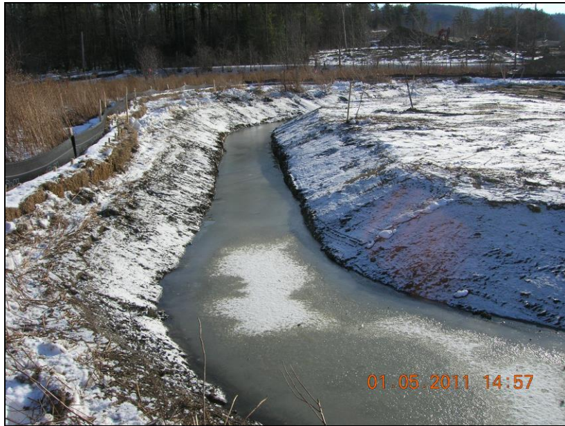
Wetland Restoration: Channel Construction January 2011
