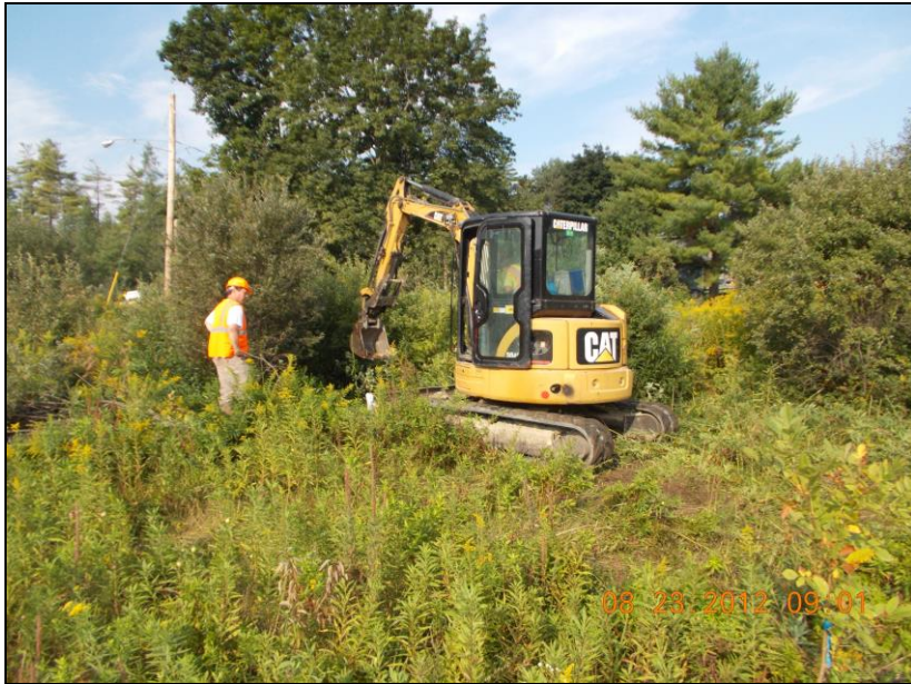
Wetland Restoration: Creating Channel Connection August 2012
