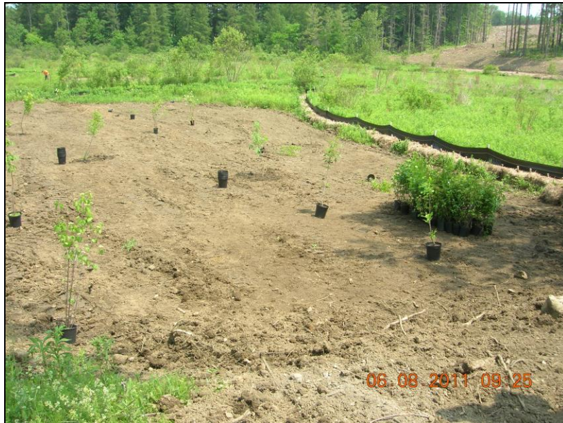
Wetland Restoration: Nursery Stock Planting June 2011
