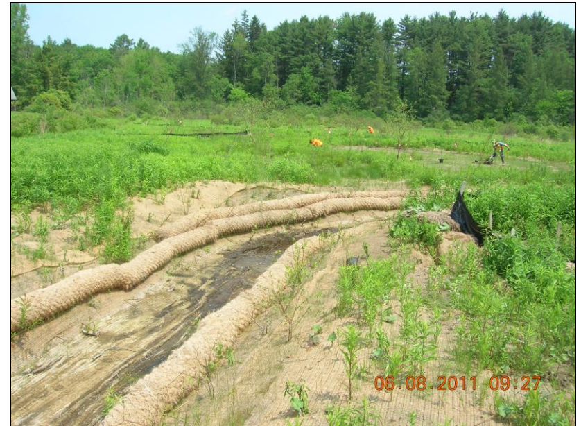
Wetland Restoration: Nursery Stock Planting June 2011
