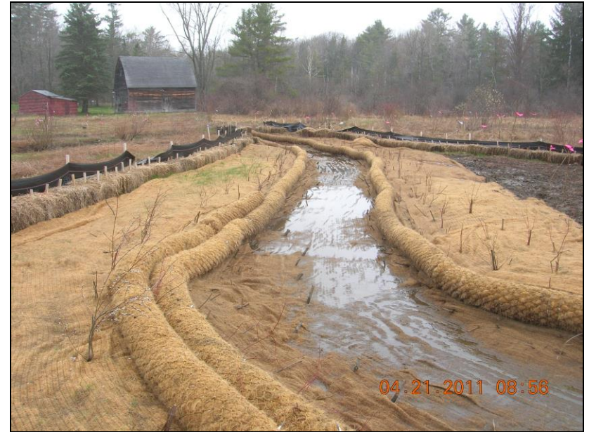
Wetland Restoration: Channel Construction/Stabilization April 2011
