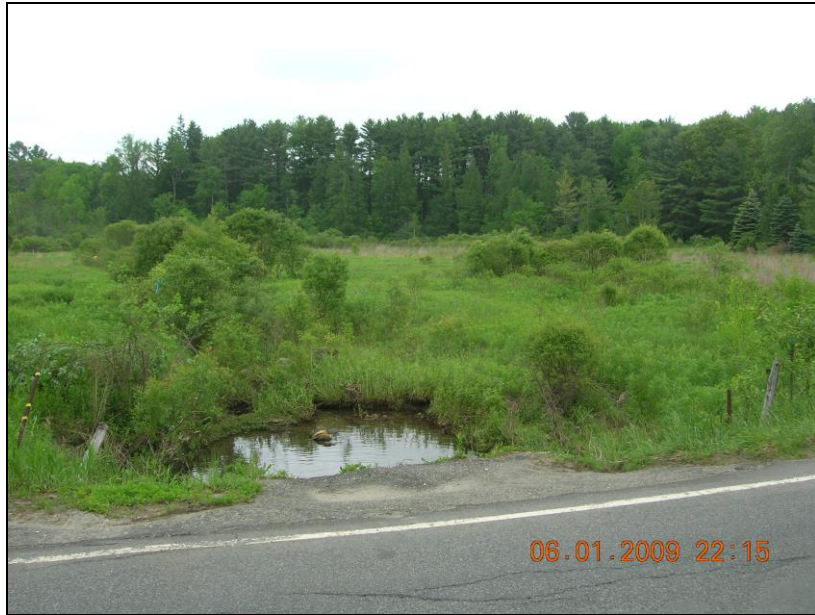
Wetland Restoration: Pre-Construction June 2009
