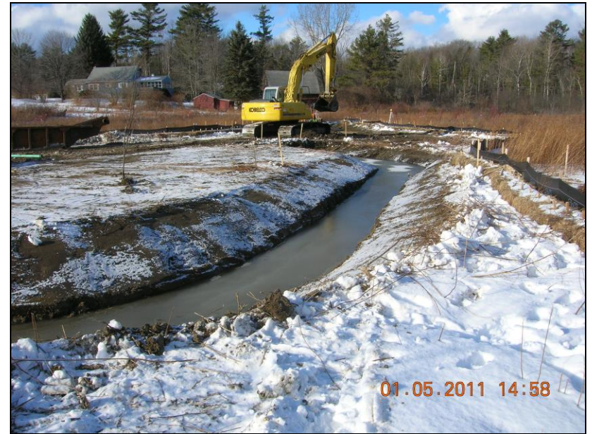
Wetland Restoration: Channel Construction January 2011
