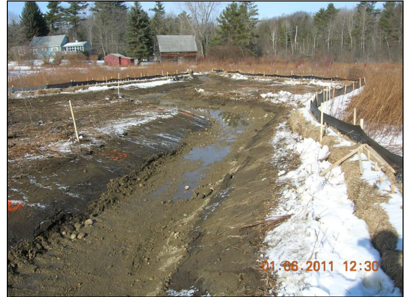
Wetland Restoration: Channel construction January 2011
